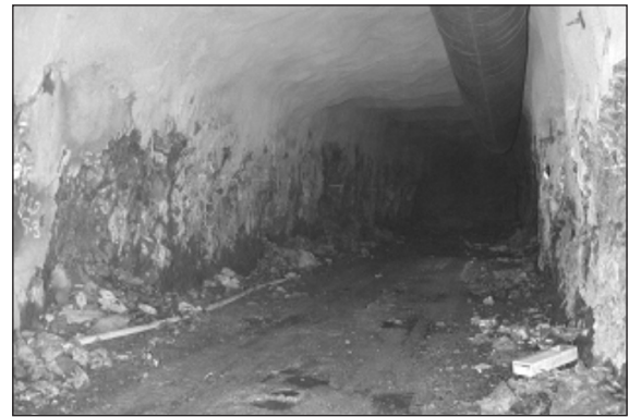
FIG. 9 Example of “minor” to “moderate” damage
