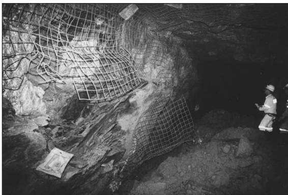
FIG. 8 Example of “moderate” to “significant” damage
