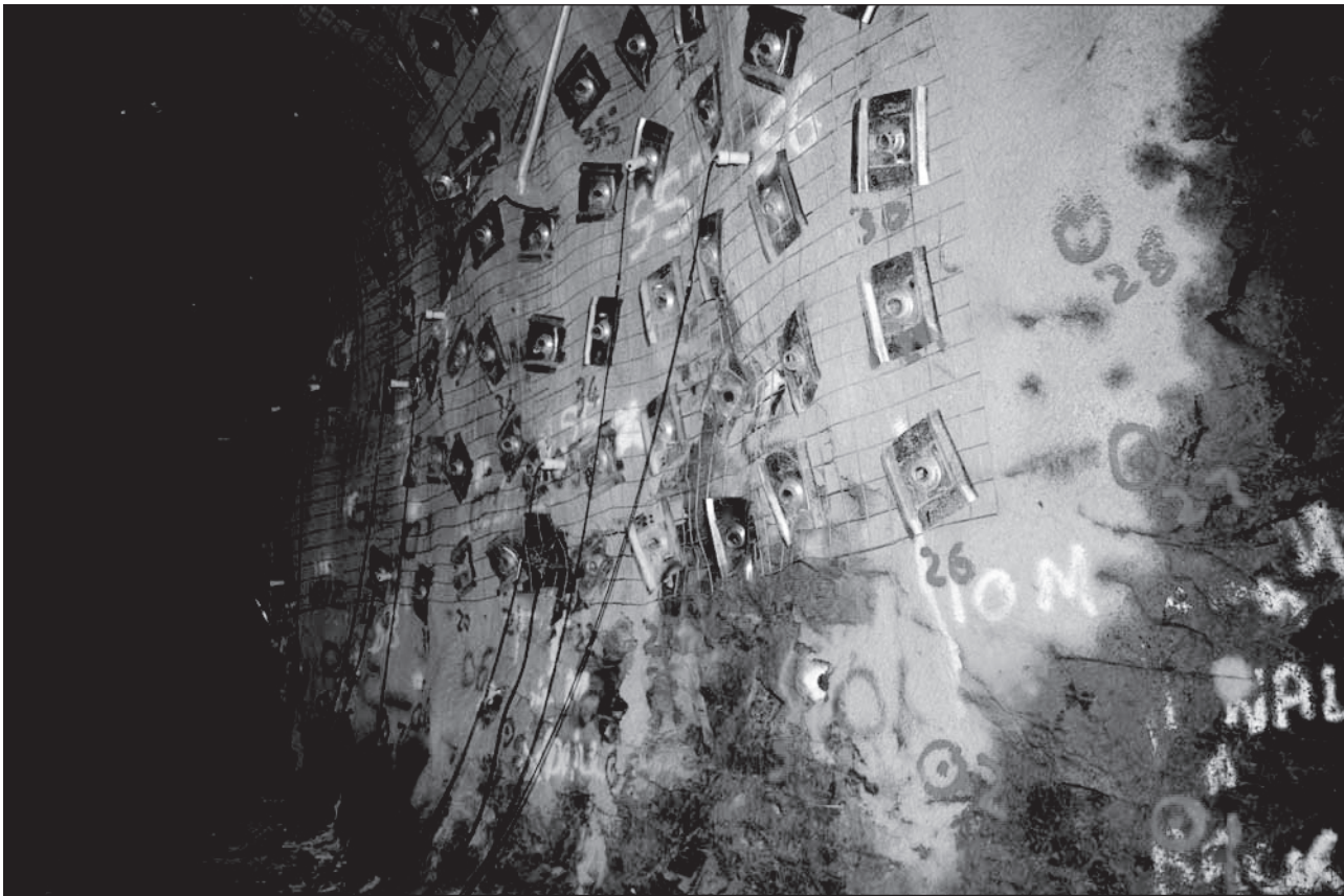
FIG. 4 Trial 1 test site
