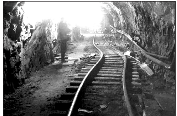
FIG. 5 Deformation of tracks in a drift as a result of mining-induced earthquake 16.04.89
