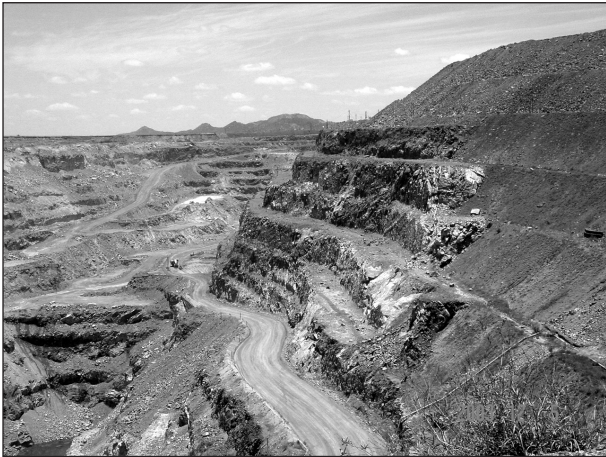
FIG. 4 The eastern slope of the Sandsloot pit, Potgietersrust Platinums Limited. A permanent microseismic system was installed here in August 2003
