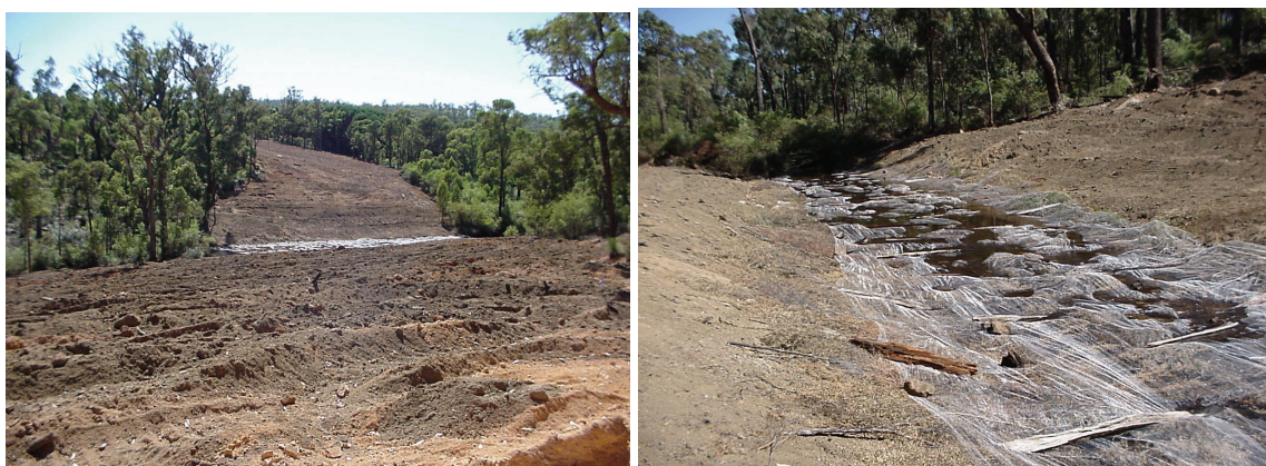
Figure 6 Rehabilitation of a haul road stream crossing: from a distance (left) and close-up (right)
