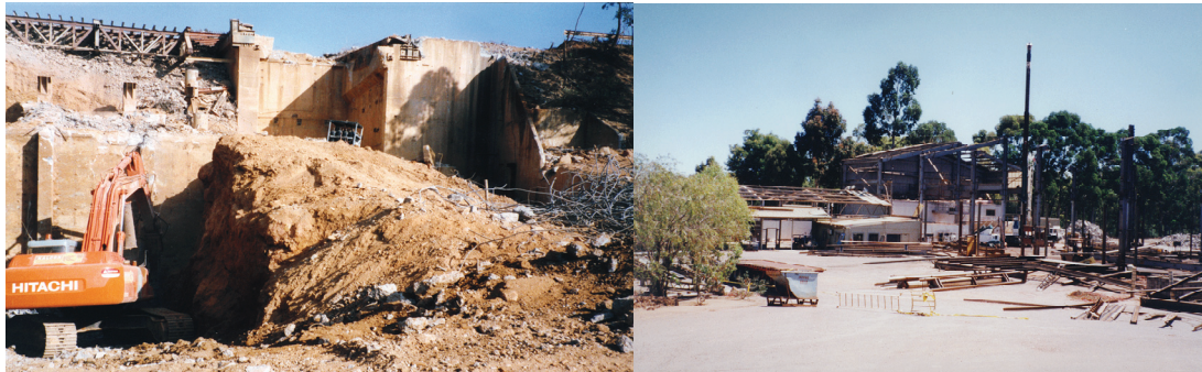
Figure 3 Removal of the crusher footings (left) and dismantling of the workshops (right)
