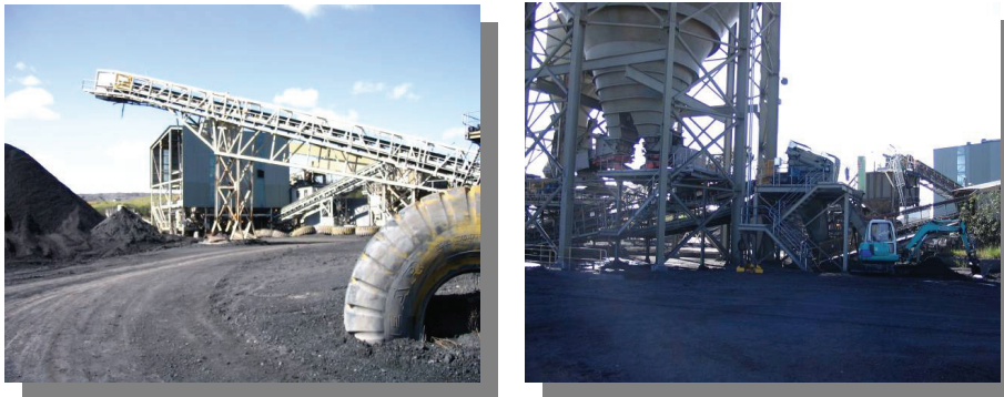
Figure 1 Infrastructure - typically this includes administration buildings, workshops, processing plants and transport infrastructure such as rail loading and roadways
