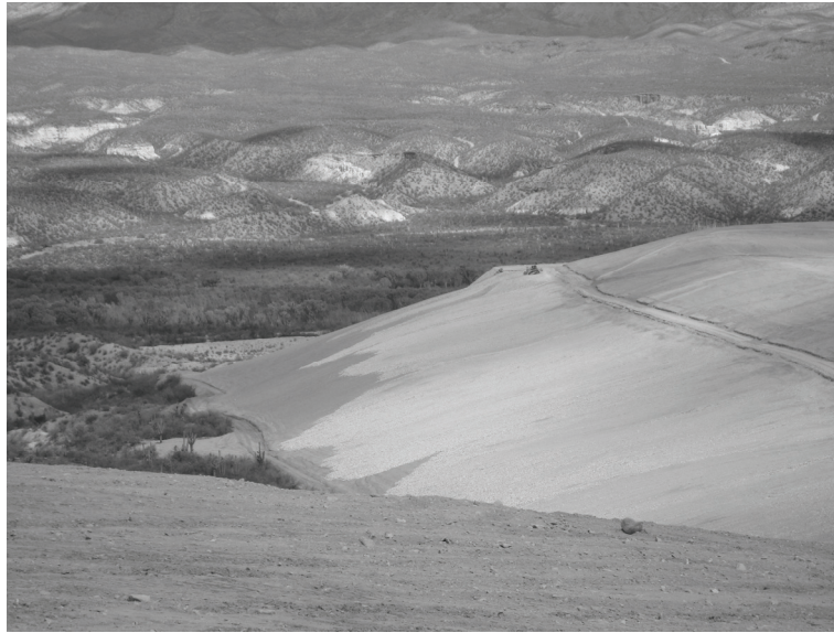
Figure 11 Construction of cover on outer tailings slope
