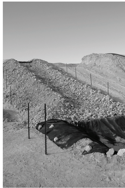
(b) rip rap
