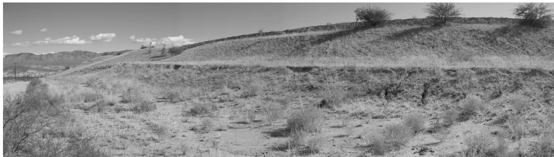
Figure 4 Revegetated fine-grained alluvium cover placed on outer slope of Dam 1 and 2 in 2002
