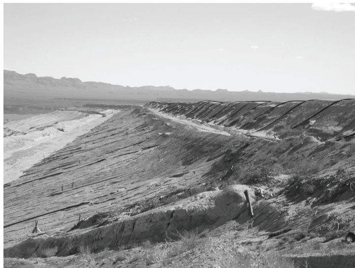
Figure 2 Unreclaimed, newer, upper bench of outer slope of 3 and 4 Dam, showing only minor erosion
