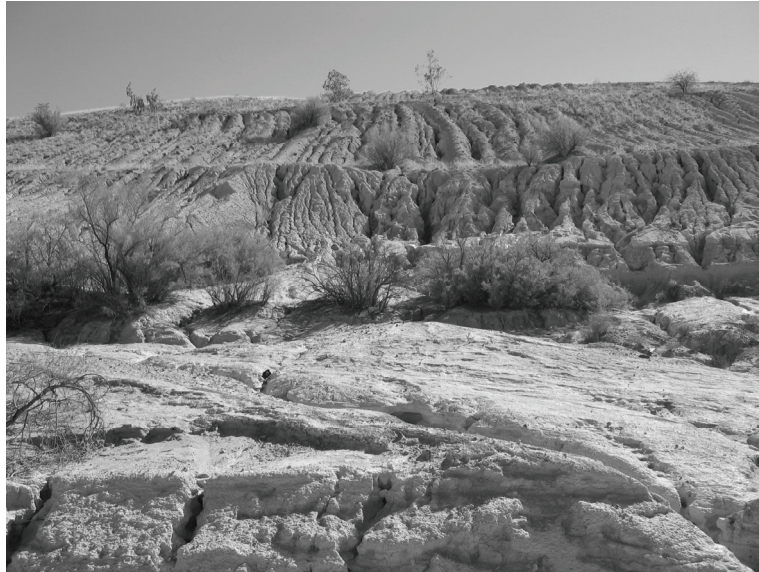
Figure 3 Unreclaimed, older, outer slope of 10 Dam, showing full-height rilling, tunnel erosion and gullying
