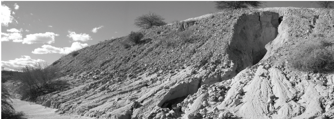
Figure 6 Poorly vegetated and gully-eroded coarse-grained alluvium cover placed on outer slope of 6 Dam in 1991
