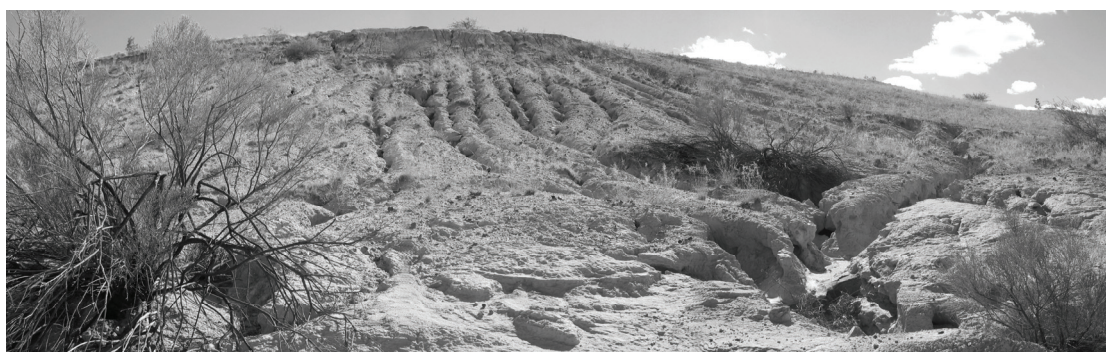
Figure 5 Now poorly vegetated and badly eroded fine-grained alluvium cover placed on outer slope of 1 and 2 Dam in 1991
