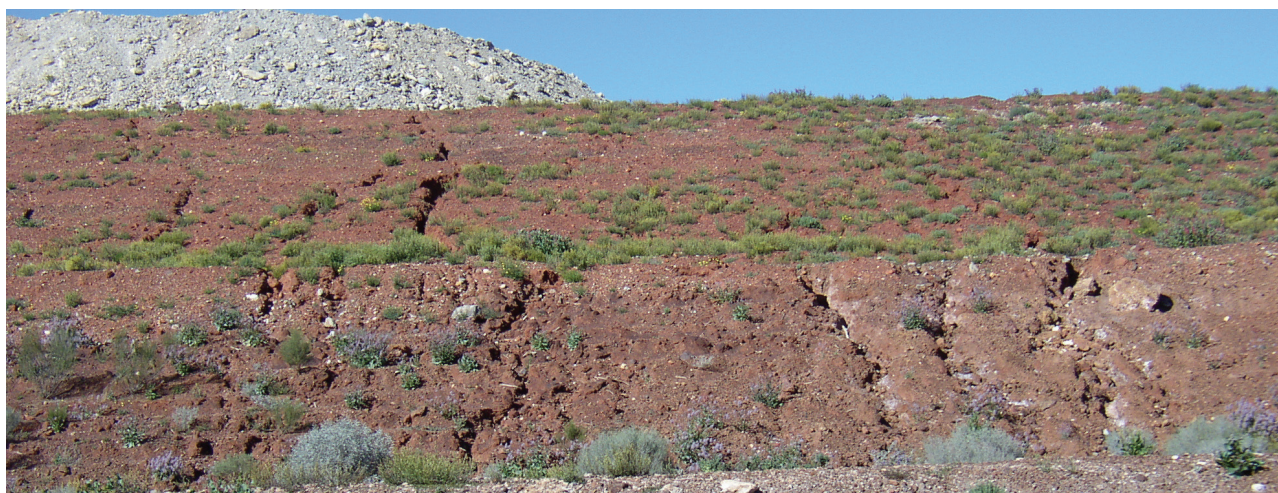
Figure 1 Typical pattern of rill and gully erosion on initial landforms at MMO
