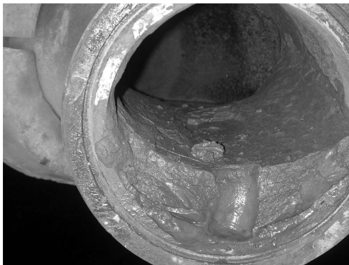
Figure 4 Laminar flow settling in paste fill pipeline
