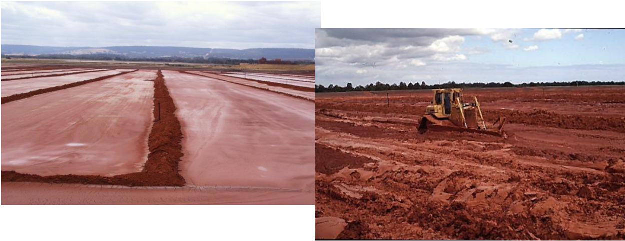
Figure 3 Spreading the slurry, and ploughing using a D6 Swamp Dozer to enhance the drying rate
