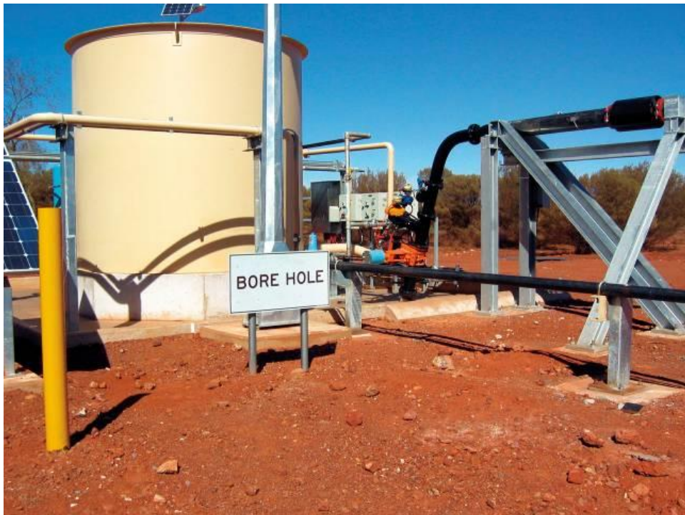
Figure 5 Drill hole for the delivery line for backfilling at Plutonic Gold Mine
