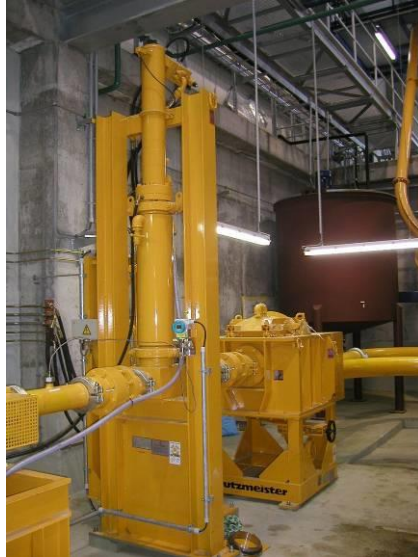
Figure 17 High pressure dampener mounted into a ZX 125 delivery line
