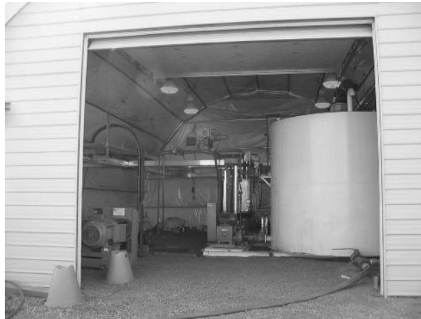
Figure 14 Interior view of full scale plant
