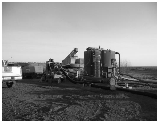
Figure 9 Lime / gypsum mix tank and MFT booster pump
