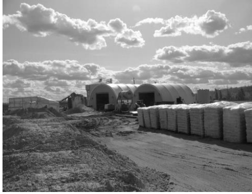
Figure 13 Exterior view of full scale plant
