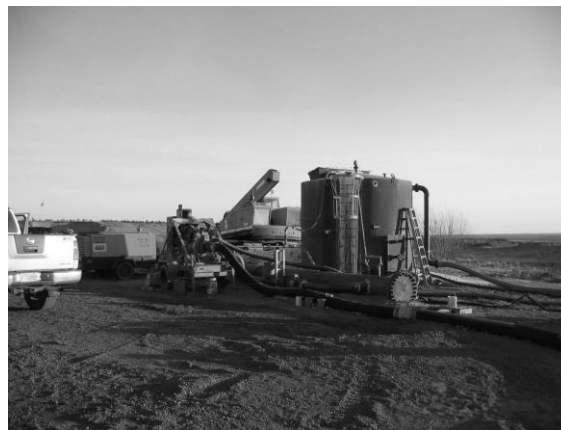
Figure 7 Loading of gypsum onto conveyor belt
