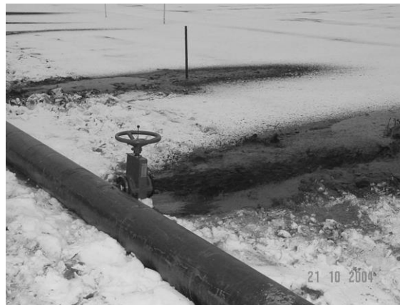
Figure 6 View of spigot pipe for deposition
