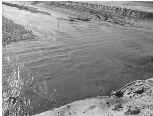
Figure 10 View of the deposition from the spigot header
