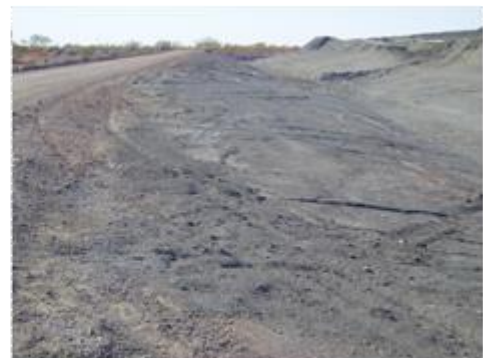
East Drain looking south
