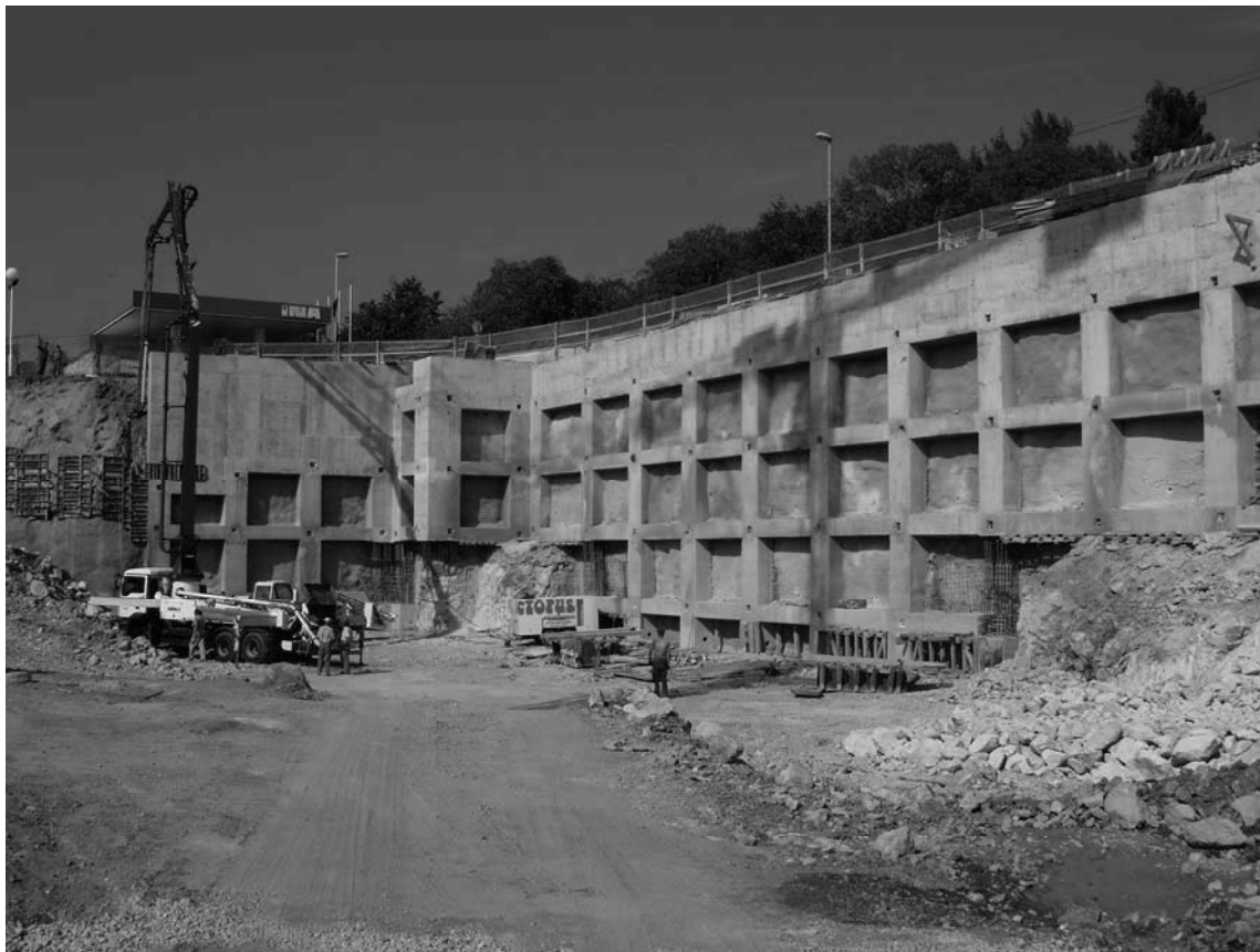
Figure 6 Reinforced concrete support construction during construction of open pit (photo Ž. Arbanas, October 2006)
