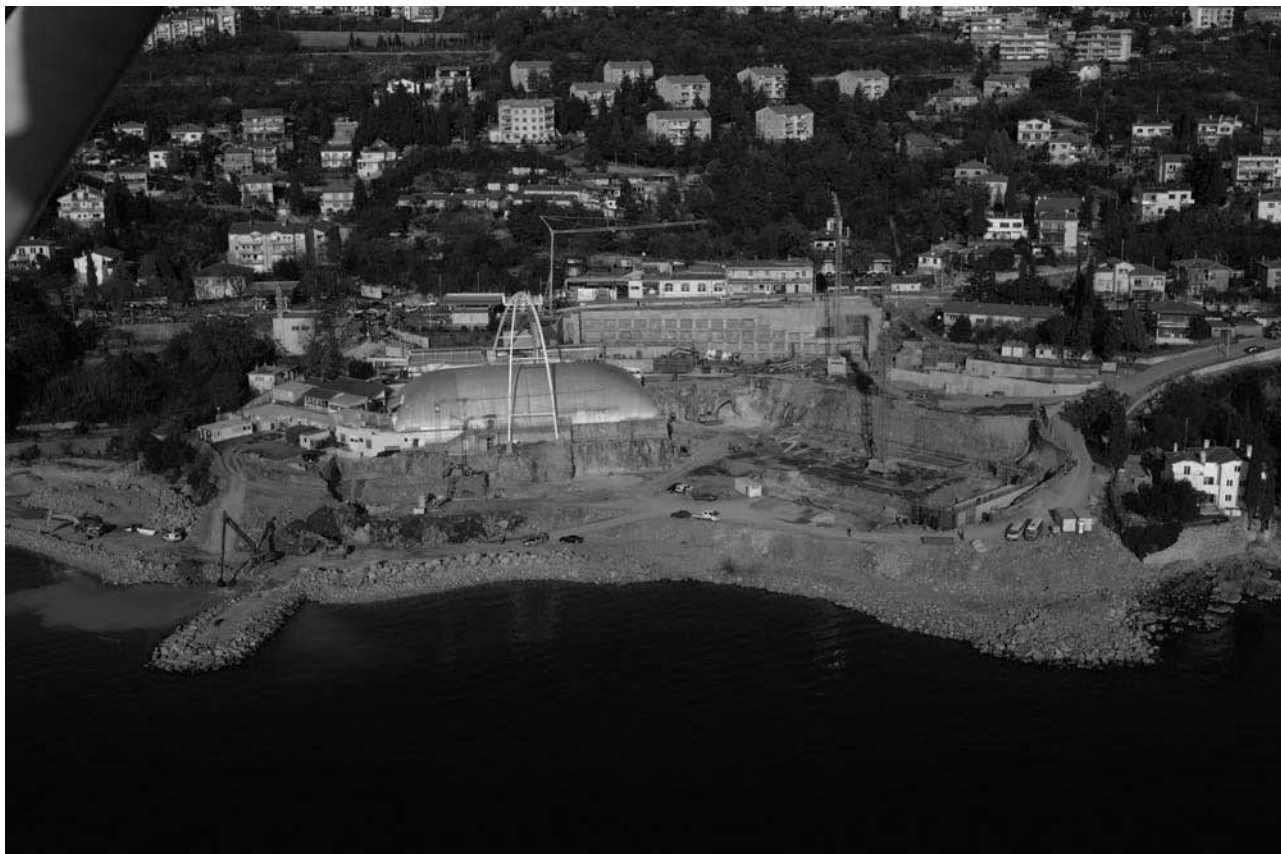
Figure 7 Aera photo of the site during work execution (photo D. Frka, December 2006)
