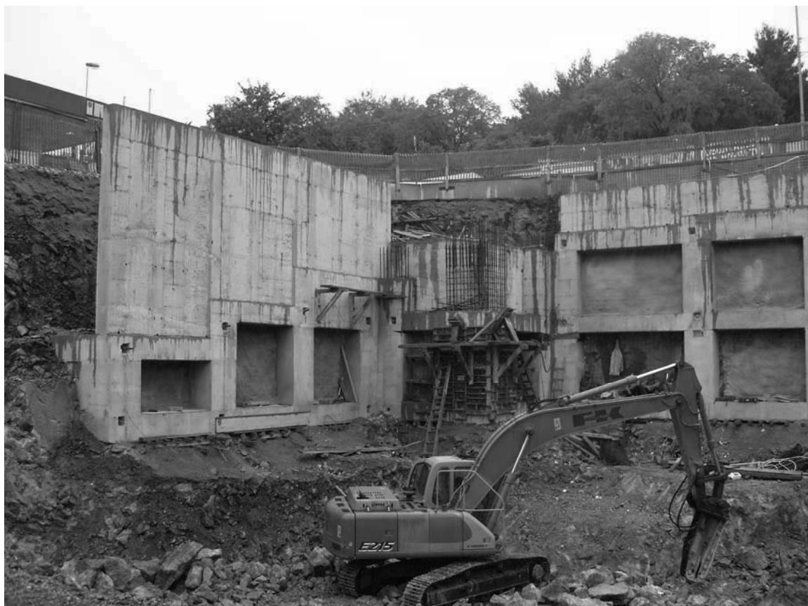
Figure 5 Reinforced concrete support construction during construction of open pit (photo courtesy Ž. Arbanas, September 2006)
