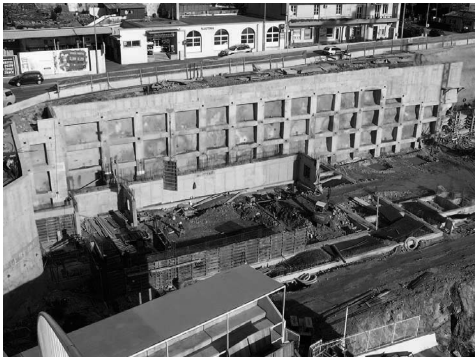
Figure 9 Photo of reinforced grid support structure on cut "North" (photo T. Pap, December 2006)
