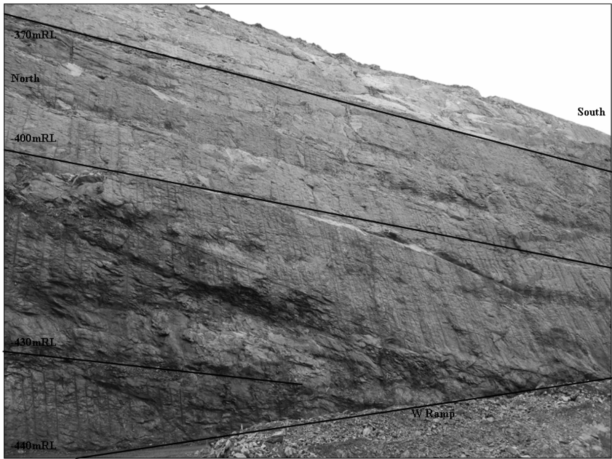
Figure 3 Trial batters on the east wall of the Fimiston Open Pit
