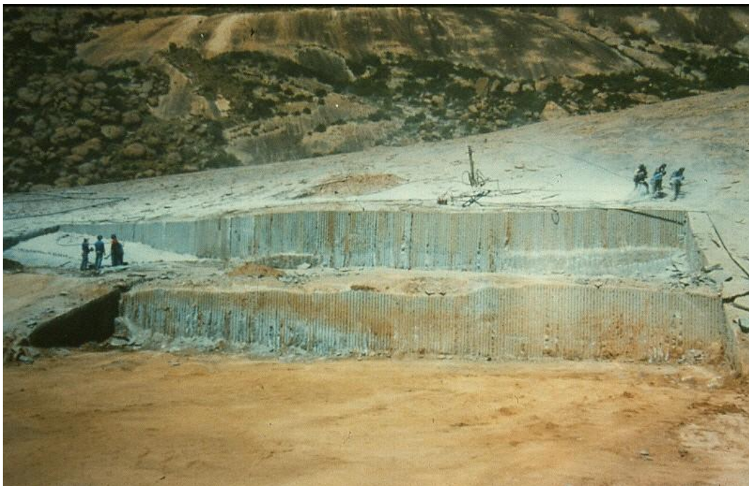
Figure 2 Extent of the quarry
