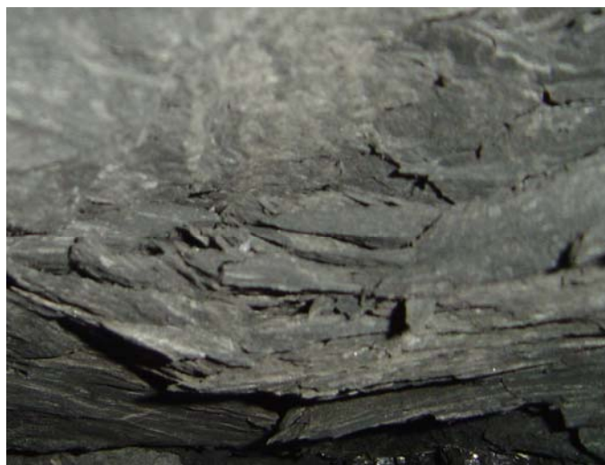
Figure 5 Stress induced fracturing ahead of a gutter. The roof gutter occurred towards the centre of a roadway
