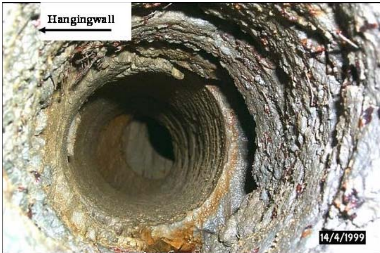
Figure 3 Shearing of 89 mm diameter blastholes in the oredrive backs (Big Bell)
