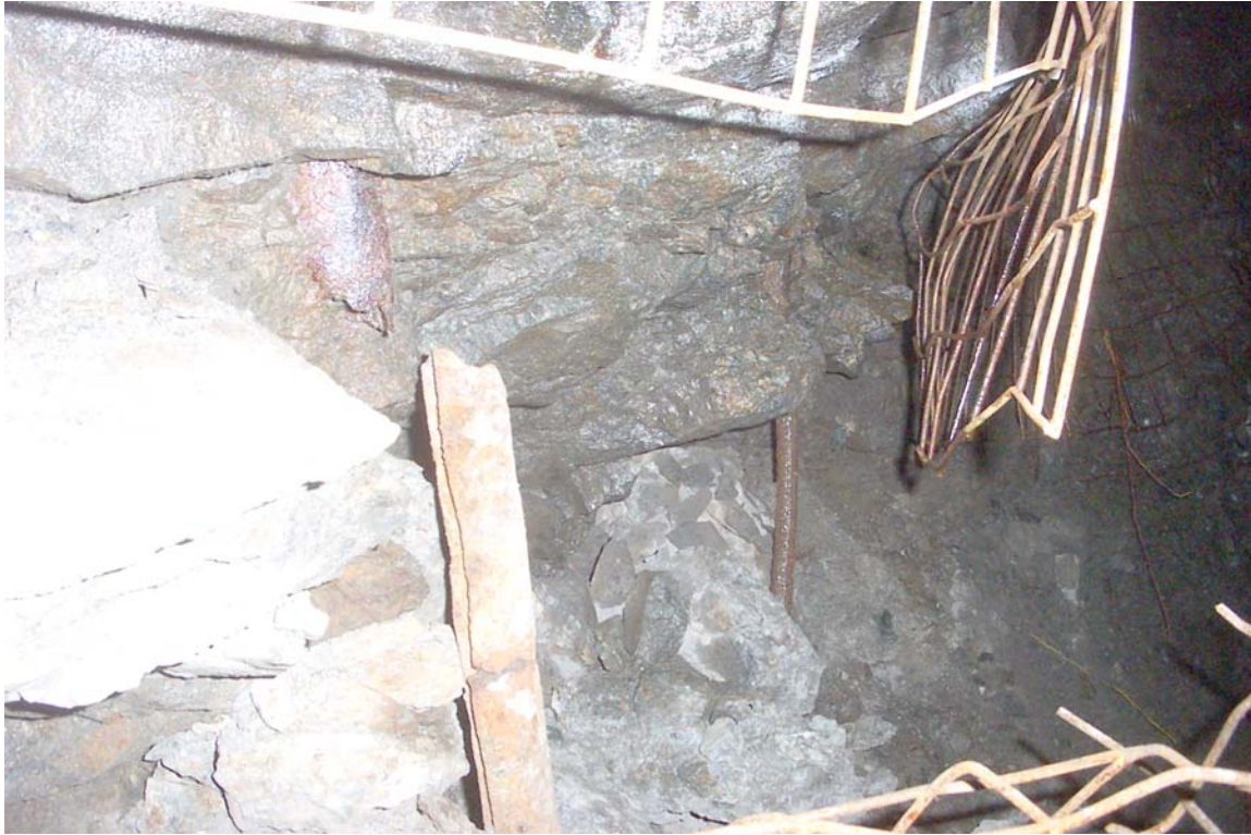
Figure 10 Sheared super swellex exposed in cut and fill mining. The rebar in the background was bent but not broken
