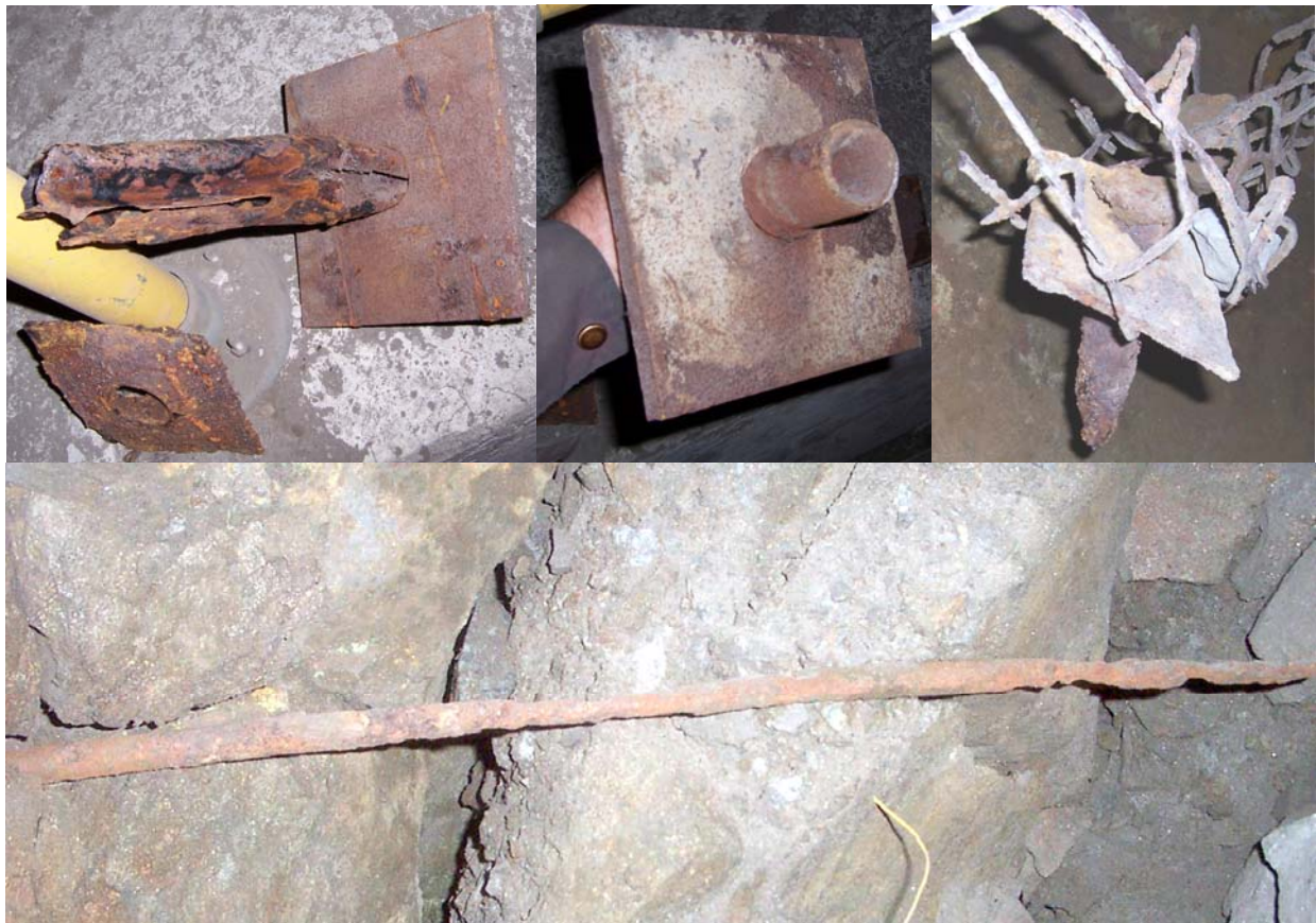
Figure 9 Upper Left – Super swellex bolt approximately 6 months old after being exposed by a small fall of ground. It was installed in a wet area in massive sulphide material (corrosive). Centre – same swellex bolt viewed from plate side with apparently only moderate corrosion. Upper right – friction set (split set) after approximately 2 years in an area with limited ventilation (high humidity). Bottom – mechanically anchored rockbolt with variable corrosion along its length (installed in massive sulphide material > 5 years, was exposed during rehab)
