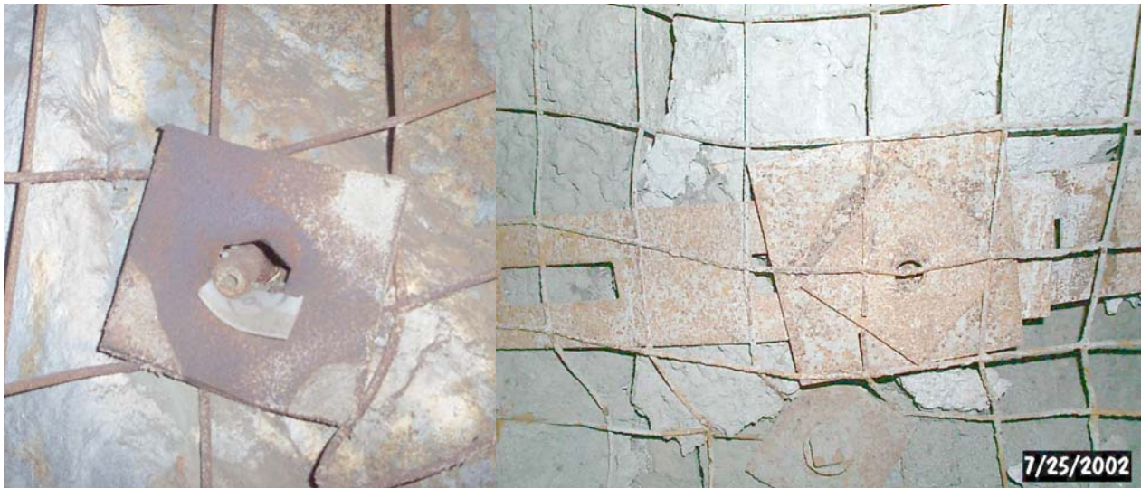
Figure 2 Left – 22 mm rebar in schist – bulking caused by schistose layers delaminating under load. Right – 20 mm rebar in meta-sediments, layered ground delaminates under high load causing heavy bulking. In this case the ground support included shotcrete covered by steel strapping and twin plates (7" x 7" with 5" x 5" plate over top). The 20 mm rebar was installed with a dome nut which popped off (rockbolt seen below rebar plates, 100 mm aperture weld mesh in both photos)
