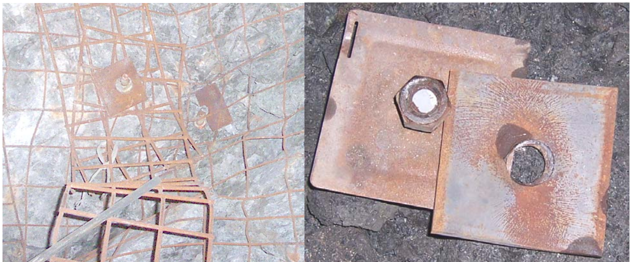
Figure 5 Left – rebar plate ripped in half immediately to the right of cone bolt (yielding tendon) over 00 gauge strap. This area experienced dynamic loading from a M n 2.6 event approximately 15 m away. Right – No.7 rebar snapped at threads. A small amount of rust can be seen on the otherwise fresh bar break probably due to eccentric loading/bending of the bar (push plate seen on bottom, rebar plate on top)
