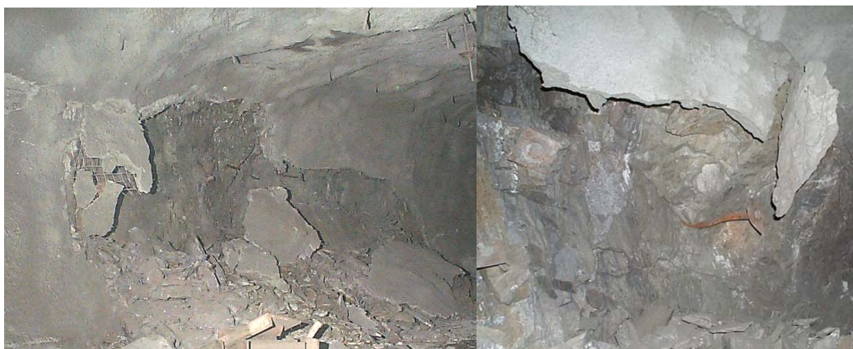
Figure 12 Shotcrete after rockbursts (two separate incidences). Both had dramix steel fibres in a prescribed thickness of 75 mm. Left photo also had No.9 gauge weld mesh in top half of wall. In both cases about 75% of the bolts were left virtually intact (mix of splitsets and No.6 rebar). In both cases the shotcrete was applied over the primary support (rebar, splitsets and screen) and thus didn't help transfer load to the tendons
