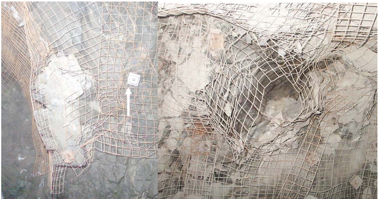
Figure 6 Left – bulking in blocky ground. Wall screen is splitting at seams; a push plate is denoted by the arrow. Right – back screen between straps and cone bolts after Mn 2.0 event approximately 10 m away (about 1.5 tonnes of loose spilled out)
