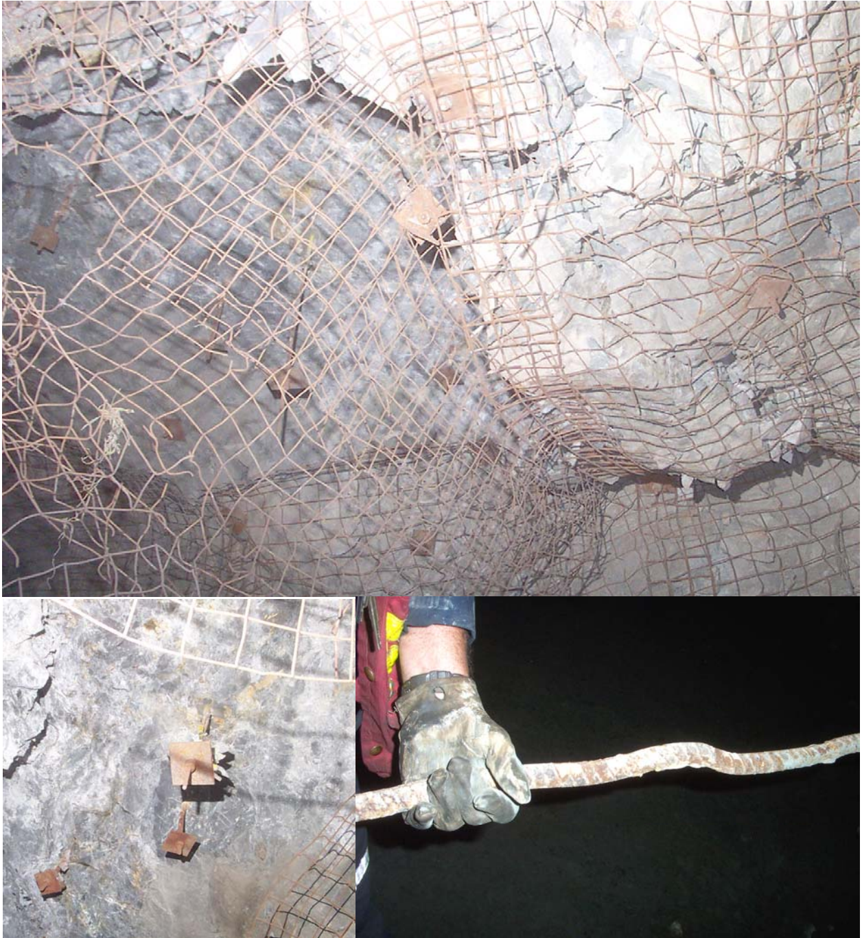
Figure 8 Back burst in blasthole overcut after floor mined out
