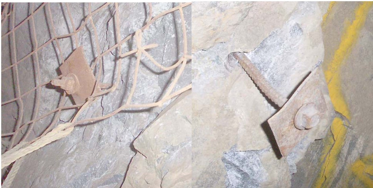
Figure 7 Left – Zero capacity bolt – mechanically anchor rockbolt in wall – plate is vertically aligned allowing minor spalling to fall out more easily due to gravity – once the plate has lost contact, the end anchored bolt is no longer supporting anything. Note also lowest wall screen can allow small material to spill out (open ended between bolts). Right – forged head rebar – spalling caused plate to lose contact (similar to left photo) but at least there is a fully bonded ripple bar in the hole still acting as ground support. The forged head arguably avoids the inherent weakness conventional rolled or cut threads cause (although forging changes steel strength) but the plate can only be held tight to the rock during installation, not tightened up later as threaded bar allows
