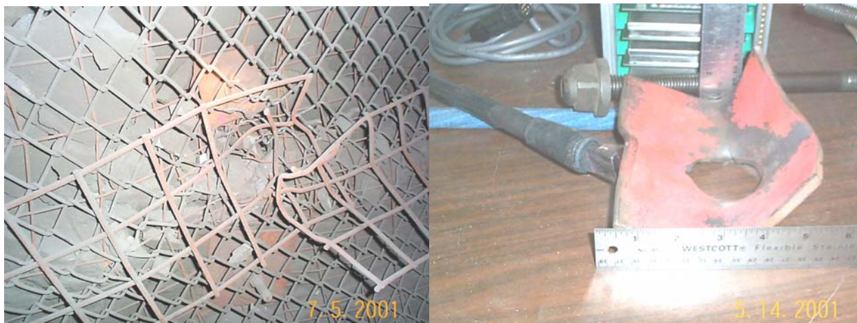
Figure 3 Modified cone-bolt plate failure. The ¼" thick plate shown in the right photo was found 6 m horizontally from the photo on the left against the opposite wall of a drawpoint. It is quite possible that the bar had seen substantial shearing and the cone wasn't able to plough. Both the cone and mixing paddle as well as the dome nut are shown in the right hand photo (similar type of dome nut as 20 mm rebar example above)
