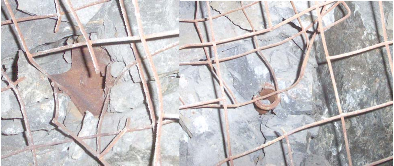
Figure 4 Left – 35 mm friction set (splitset style bolt) with folded plate and broken No. 7 gauge mesh strands (wire strand capacity about 0.9 t, 4.5 mm diameter). Right – same wall – friction set with plate torn off. Mesh strands also broken. A slip plane can be seen in right half of photo. This chloritised structure caused localised movement on the wall, pinching the bolts not allowing them to yield. Mesh is 100 mm aperture for scale. Bolt length is 1.8
