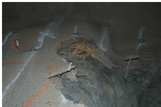
Figure 12 Ejection of Fibrecrete and Split Sets left protruding at the Darlot Walters 1240 Access test site. Note the section of mesh reinforced Fibrecrete higher in the photo suffered far less damage
