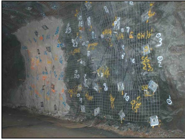
Figure 9 Completed test wall setup from Mt Charlotte, shown prior to the first blast. The numbered circles are Sirovision control points. Surface mounted geophones connected by coaxial cable are attached to the test wall surface at various locations
