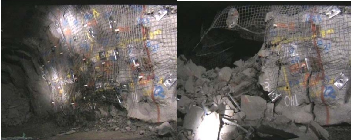
Figure 10 Before and after shots from the digital video camera at the Longshaft Rhondo North Access site. Ground support systems tested were “Split Sets and Mesh” and “Widely Spaced Split Sets and Mesh”
