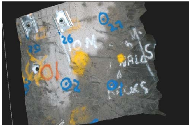
Figure 6 A three-dimensional image generated from the point cloud in Figure 5 and digital image in Figure 4
