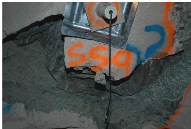
Figure 11 From Mt Charlotte 1155 Access – ejection of rock supported with Masterseal 845A TSL around Split Set plates. A rockbolt mounted geophone is visible
