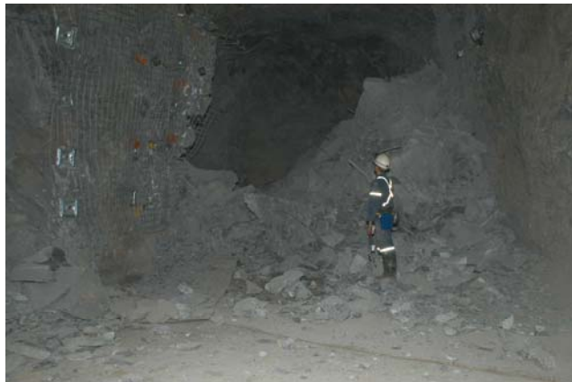
Figure 14 After the 2 nd blast at the St George site. The system in the foreground (Split Sets and Mesh with Cone Bolts) mostly survived however the other system (Split Sets and Tunnelguard TSL with Cone Bolts) was completely destroyed
