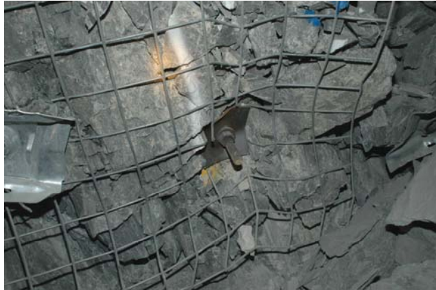
Figure 13 Moderate damage to the Split Sets and Mesh with Cone Bolts test section at the St George 8 Level Stockpile site. Severe bulking of mesh was observed and the small Cone Bolt plate has cut the mesh
