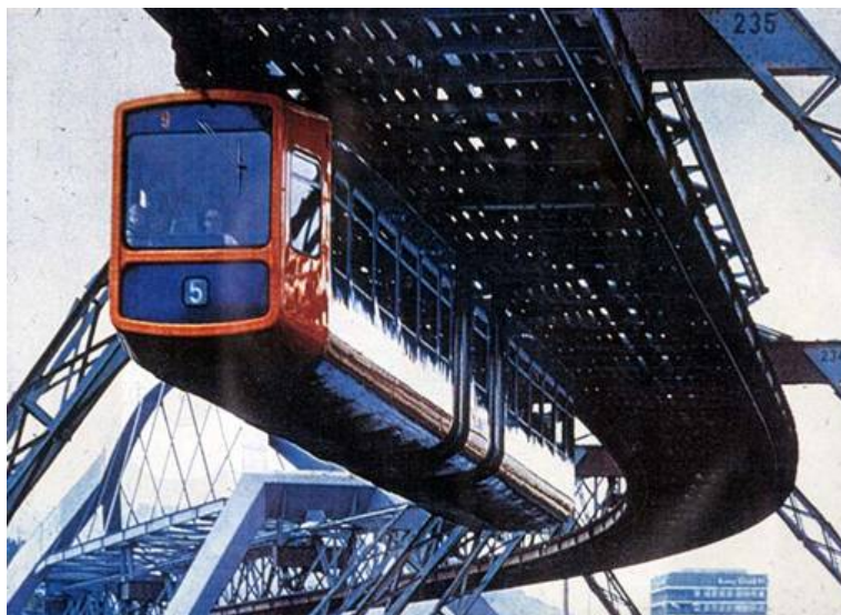
Figure 2 The monorail at Wuppertal
