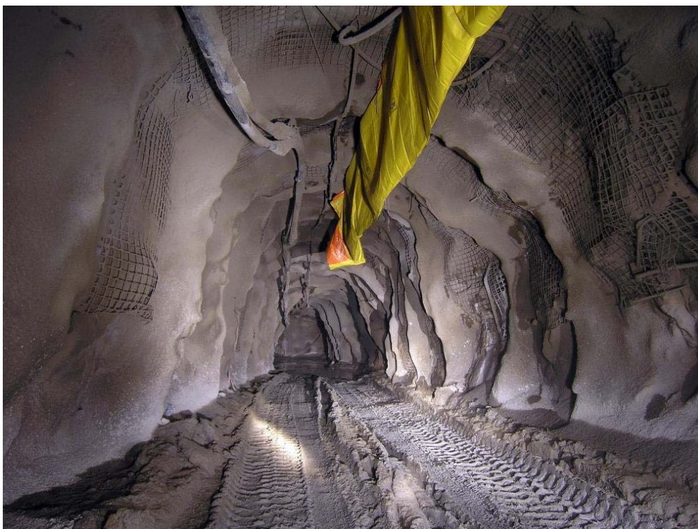
Figure 6 Fibrecrete arches on 475 m level
