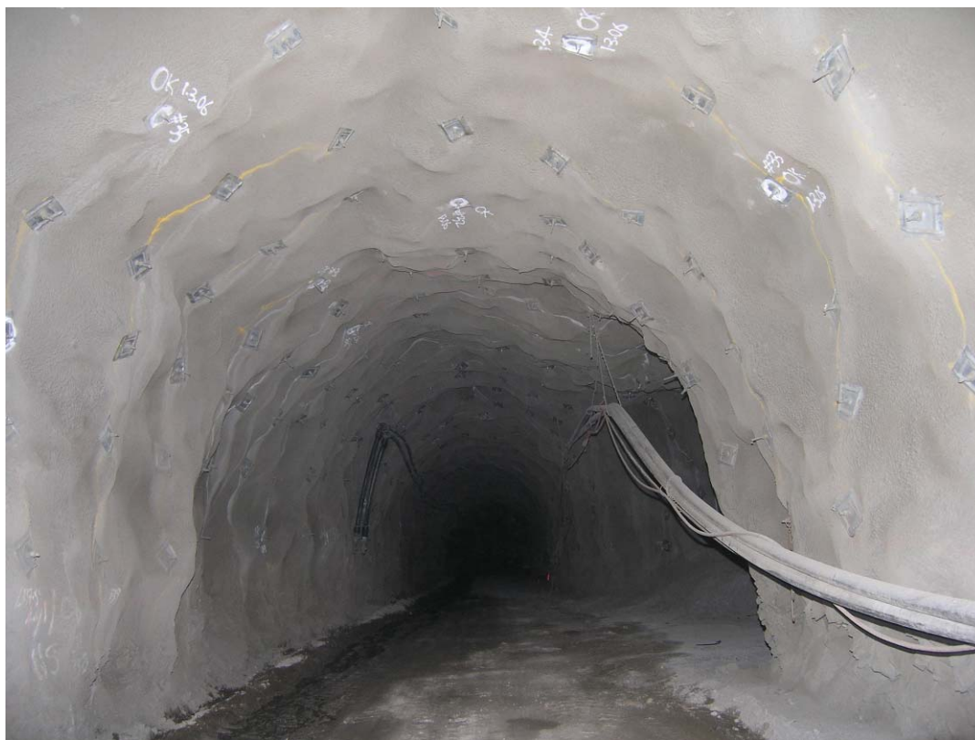
Figure 4 Decline photo after application of Fibrecrete surface support and Posi4bolting
