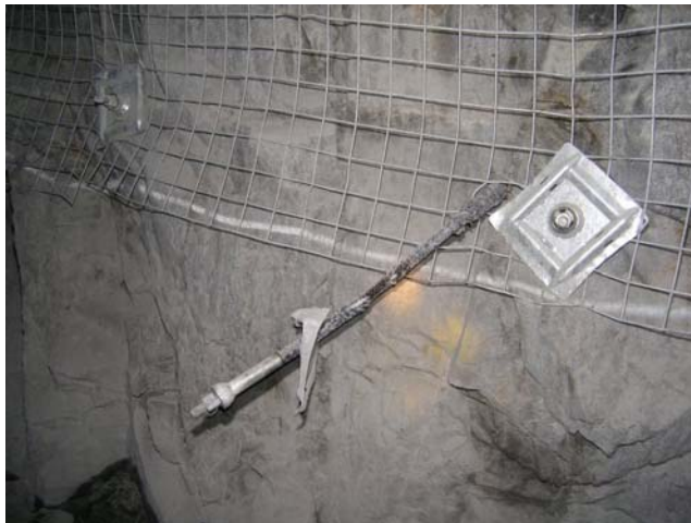
Figure 8 Damage poly grouting sleeve on a hybrid bolt
