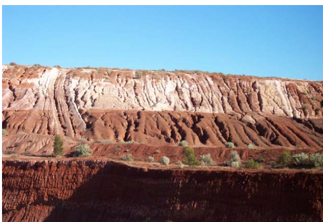
Figure 2 Surface water damage to dump faces (left); and facility for ongoing treatment of dump runoff (right)
