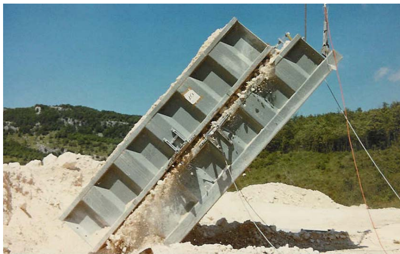
Figure 4 In situ 5 m long rockfill tilt test being performed during dam construction in Italy (Strøm, 1987)
