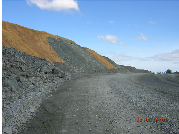
Figure 14 Clay facing under construction
