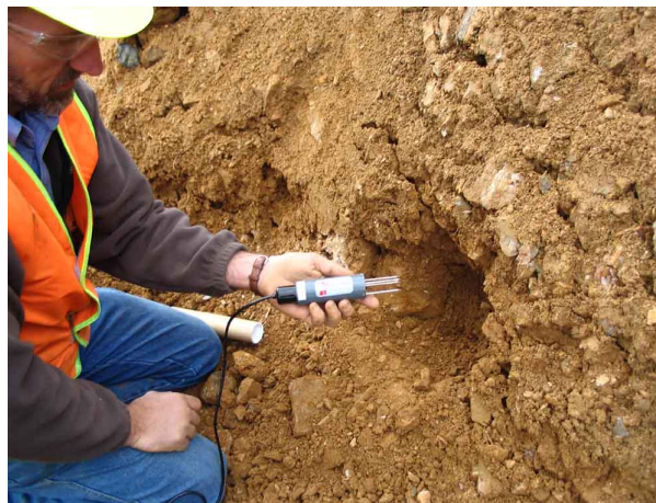
Figure 16 Installing the Theta probe moisture monitors
