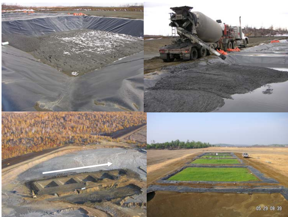
Figure 9 Sequence showing the construction of the INCO lysimeter experiment
