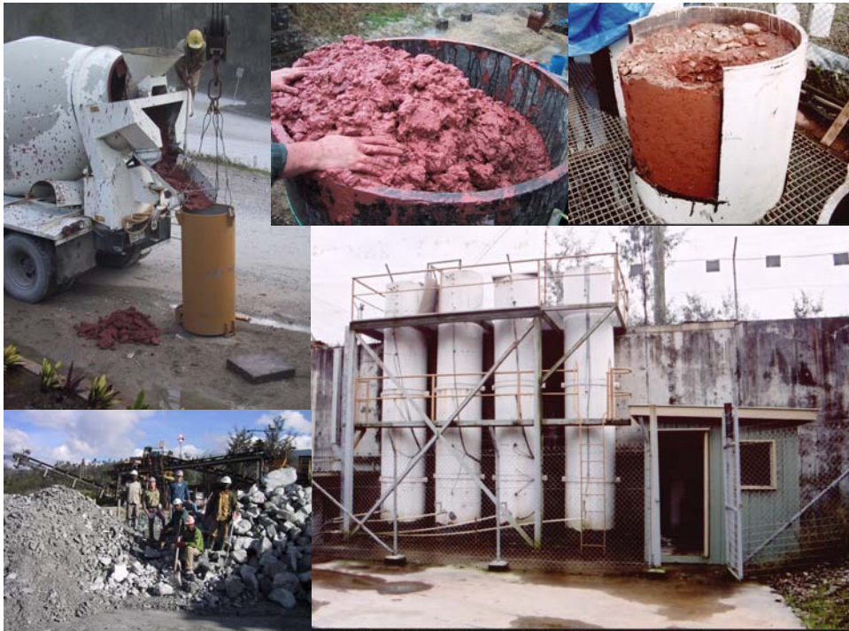
Figure 2 Construction of the meso-scale column experiment at Porgera mine
