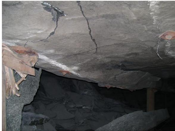
**Figure 3** Fall of ground in the ledge of Panel 4S (Position B, Figure 8). Observations indicate that this fall appears to have been caused by shear failure in the hangingwall next to the abutment on this ledge
