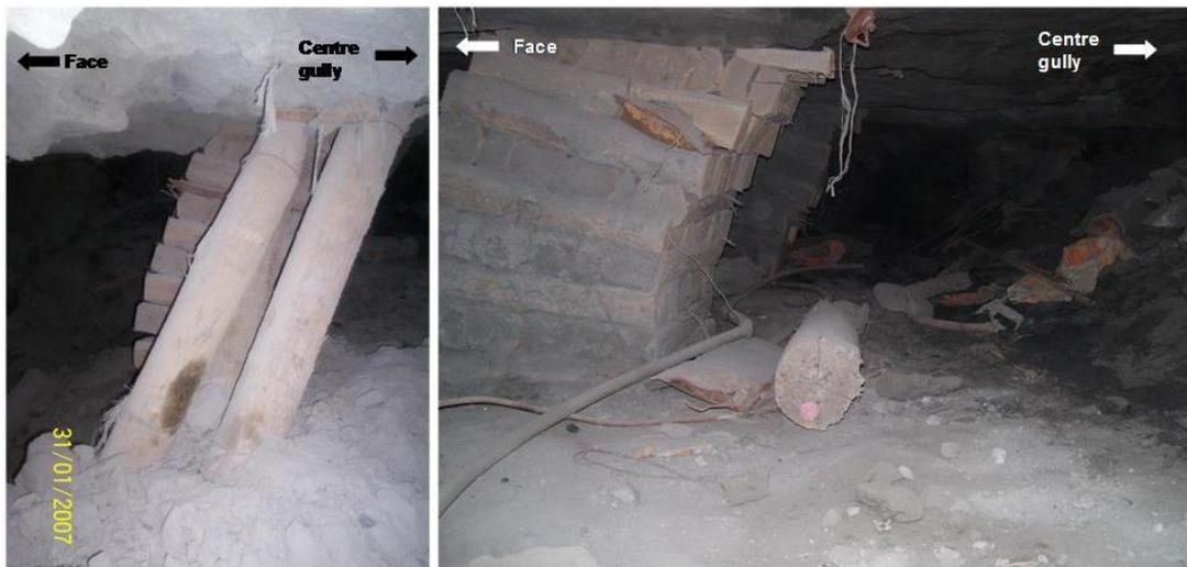
**Figure 2** Strong ride component observed in the back area of Panel 4N close to the centre gully (Position A, Figure 1). The sense of the ride component is such that the hangingwall moved towards the centre gully
