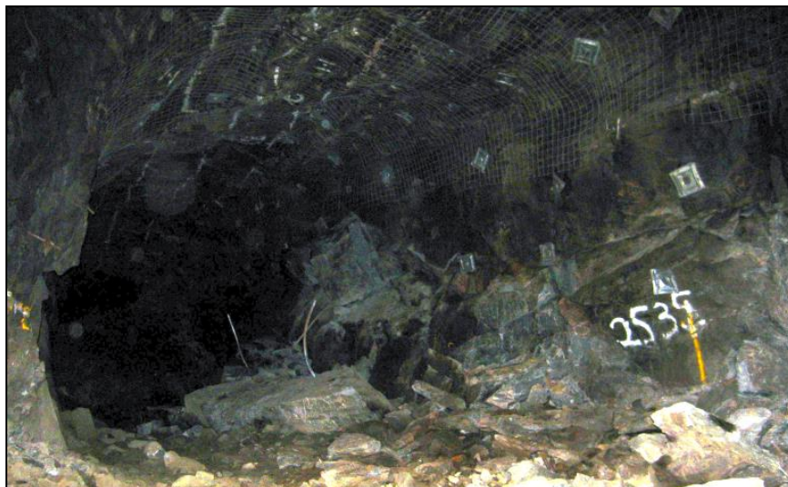
Figure 5 Damage in the ROB5 2535 drive associated with a Richter magnitude 1.7 seismic event following a blast on 4 June 2007
