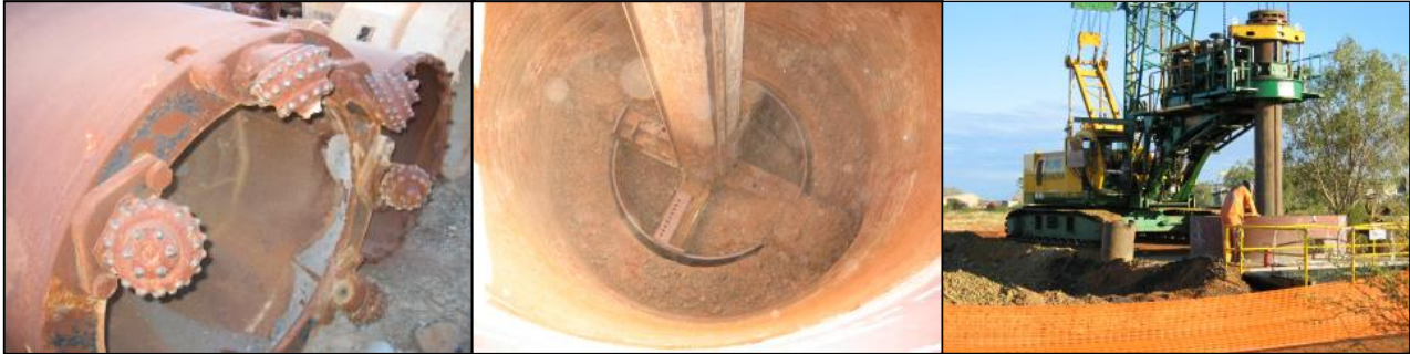
Figure 3 Large diameter piling technology
