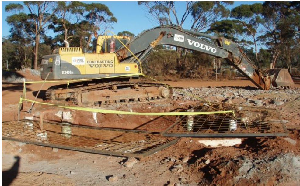
Figure 8 South raisebore site during excavation for the surface pad. The tops of several of the bored piles are visible in the walls of the excavation
