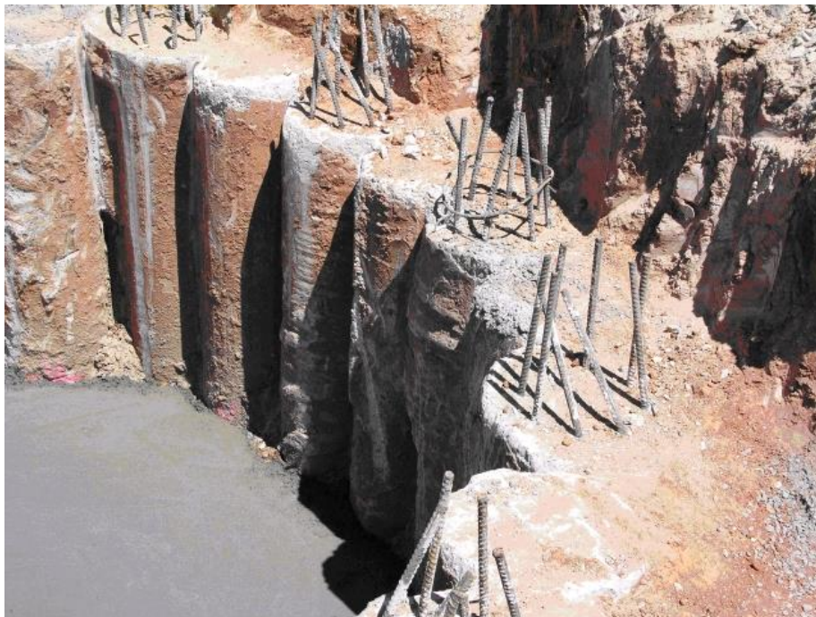
Figure 4 A ring of contiguous bored piles forming a curtain at another mine site
