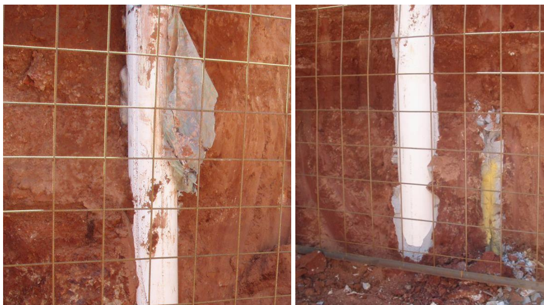
Figure 10 Some of the bored grouted piles intersected in the surface pad excavation, showing grout filling the sidewall voids created during the boring of the RC holes
