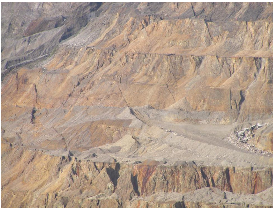
Figure 12 Side View of failure area, with toppling towards LHS (benches are 15 m high)
