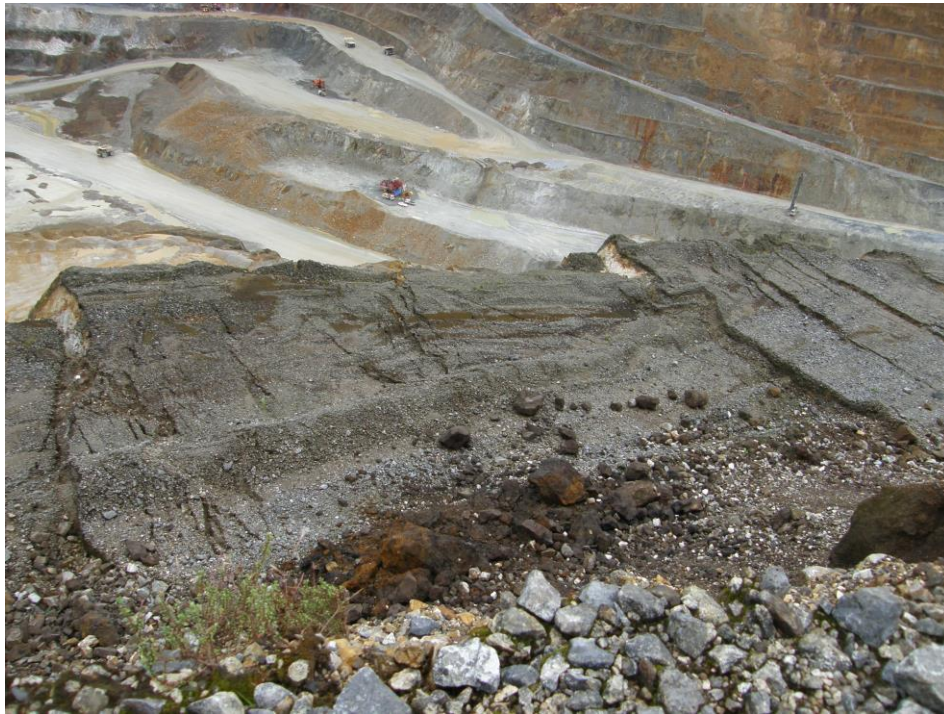
Figure 11 1.5 m step-up on defects: toppling failure direction is towards RHS (8 m wide bench)
