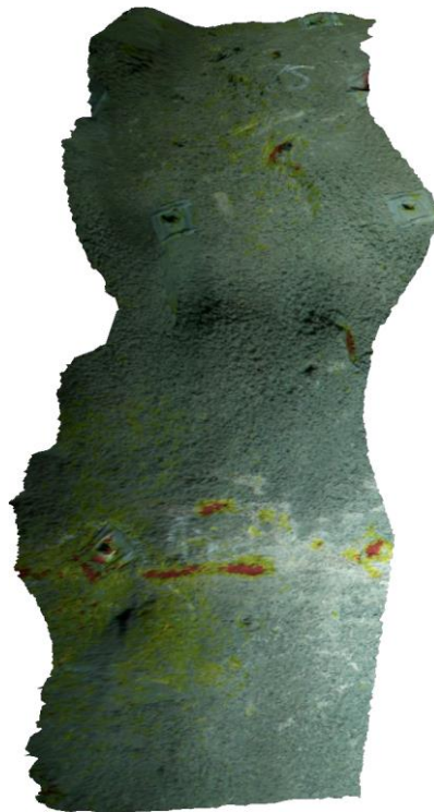
Figure 9 Accuracy check (note damage caused by bogger)
