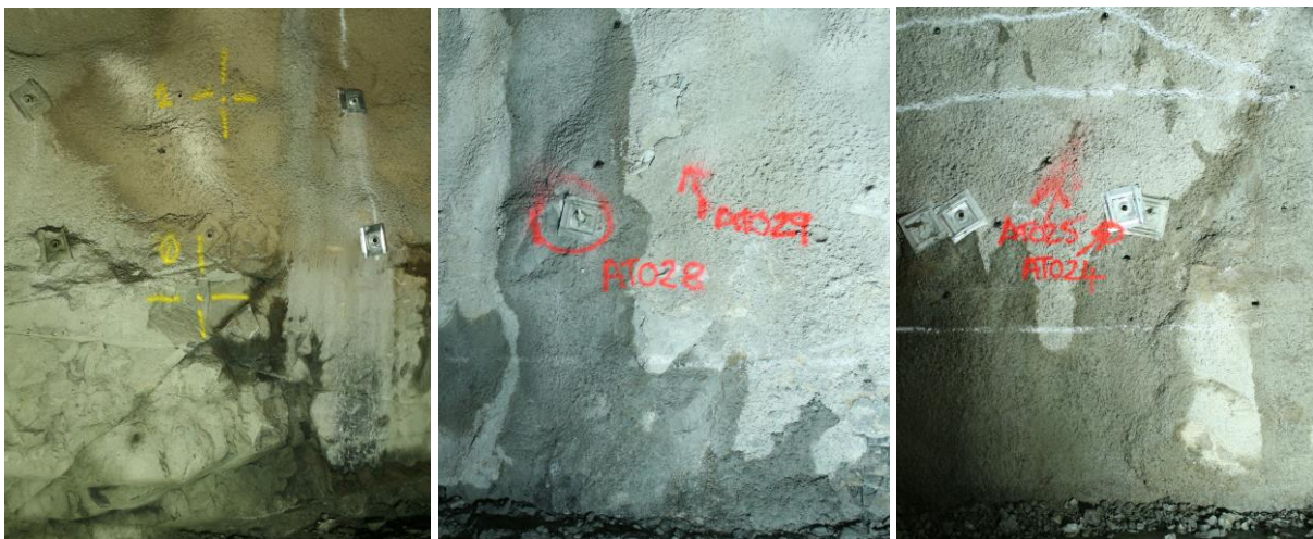
Figure 2 Control points painted on the wall, using existing gewi bolt heads and plate corners
