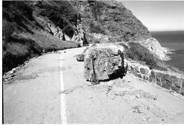
Figure 3 A 2–3 m 3 peninsula sandstone block at rest on the Drive
