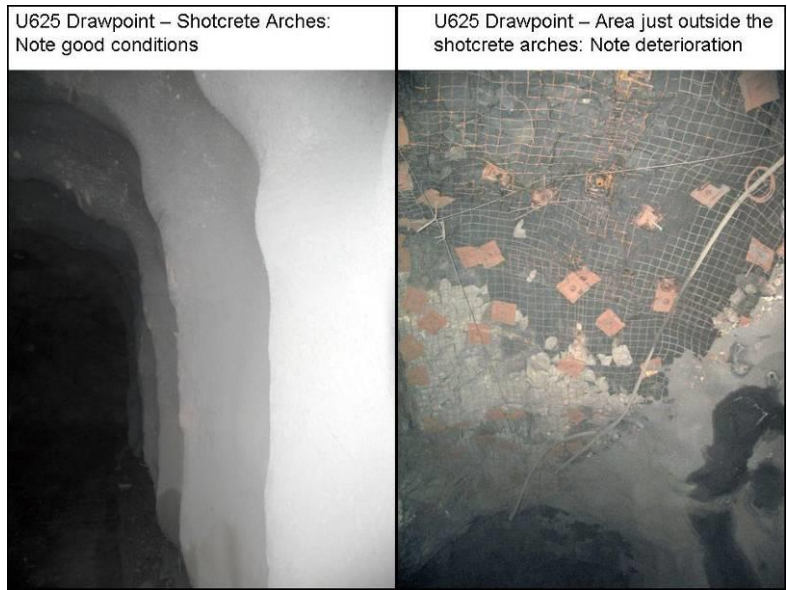
Figure 13 Photos comparing shotcrete arches versus conventional support
