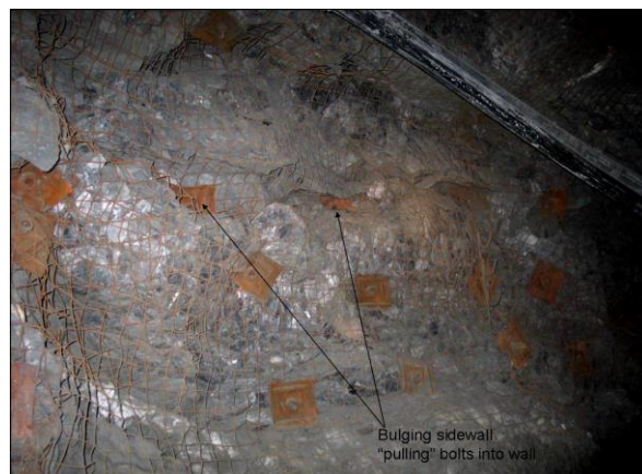
Figure 11 29E Level drive deformation. Note cable bolt plates ‘pulled in’ as the rock mass deforms around the solid anchored steel
