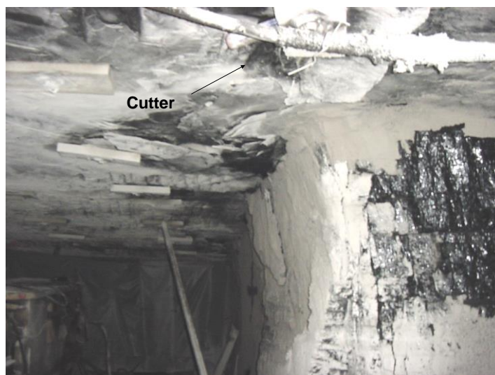
Figure 6 The onset of a cutter into the roof against the pillar rib
