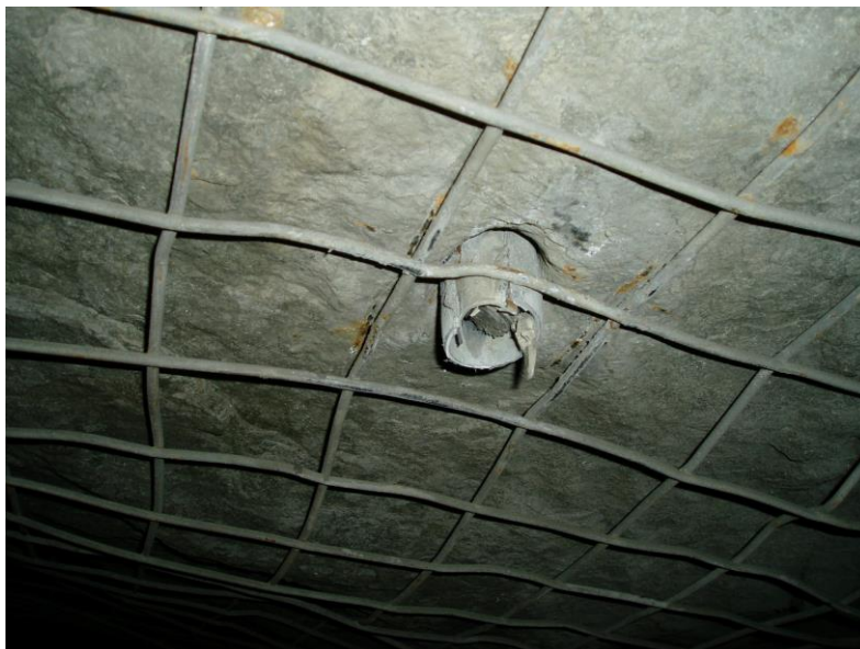
Figure 8 Remnant of a Stiff Split Set in a back hole after pull testing to 200 kN
