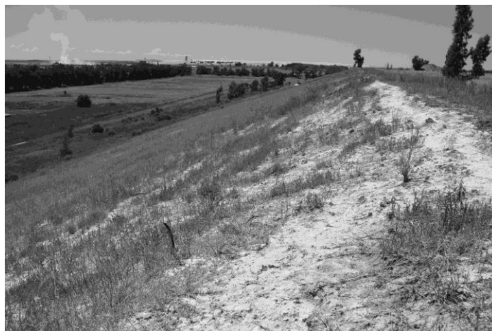
Figure 2 A TSF external wall adjusted to a 16^\circ slope, with an abundant grass cover still remaining 10 years after planting. Note also that runoff from the top surface over the external slope has not occurred
