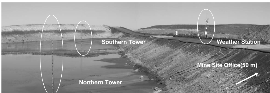
Figure 3 Commencement of tailings deposition into the trial cell
