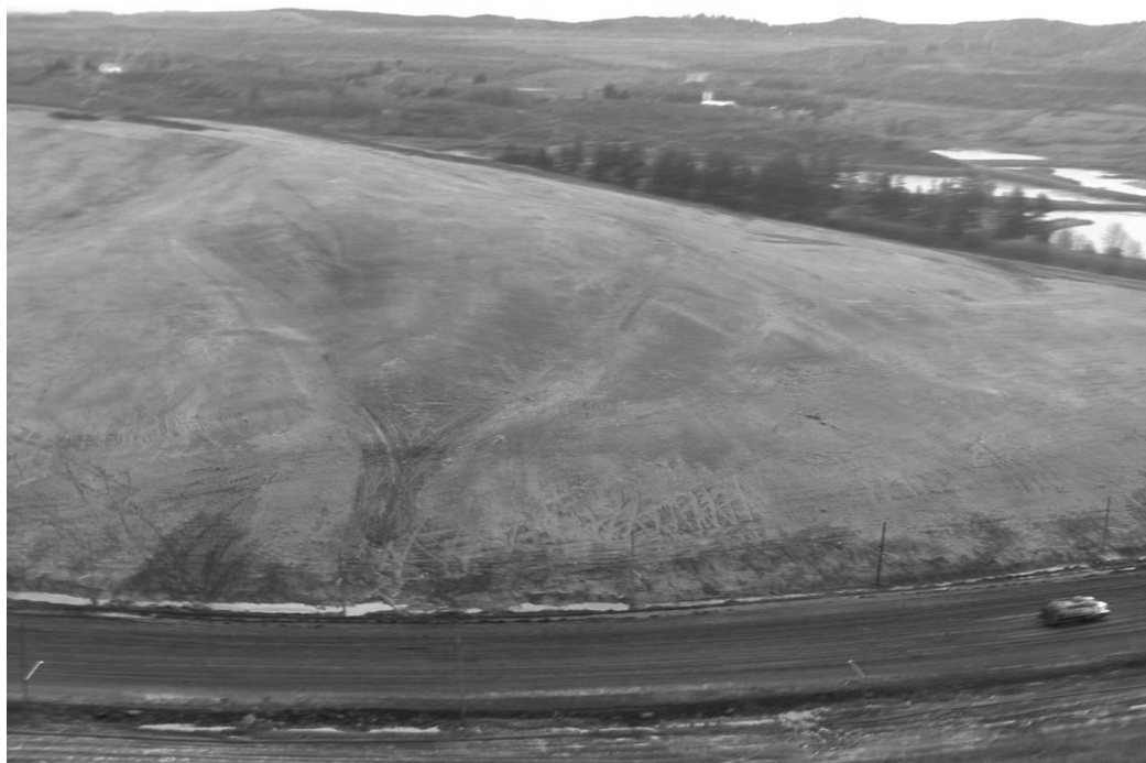
Figure 3 Vegetated swales built into an overburden waste dump at a coal mine in Washington State
