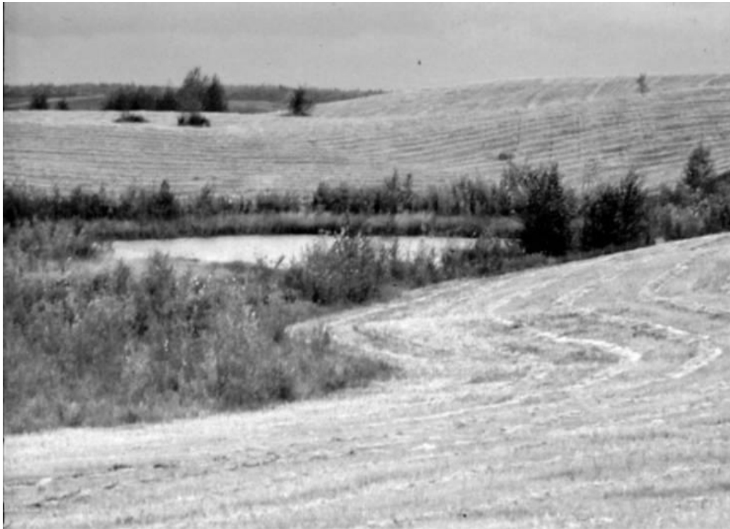
Figure 2 Irregular topography built into an overburden waste dump in East-Central Alberta
