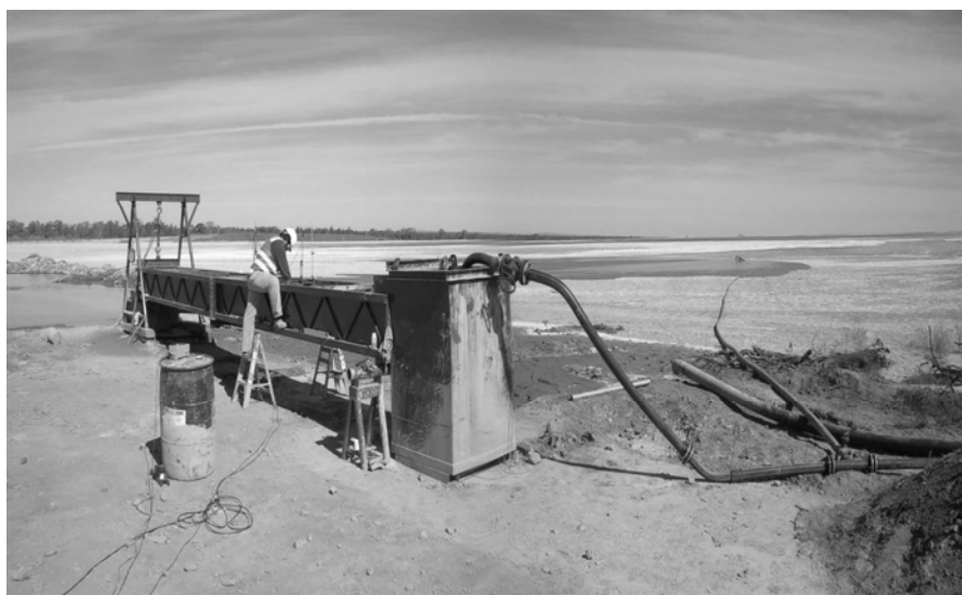
Figure 6 Large scale flume used during the Peak and Sunrise Dam experimental work
