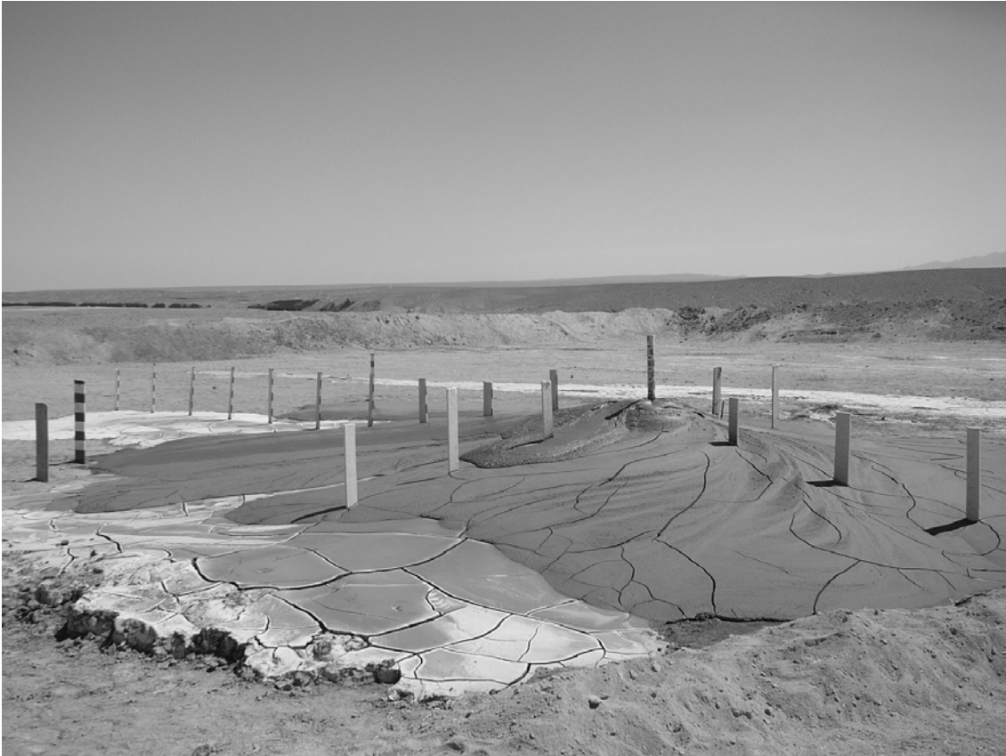
Figure 2 Thickened tailings showing early cracking
