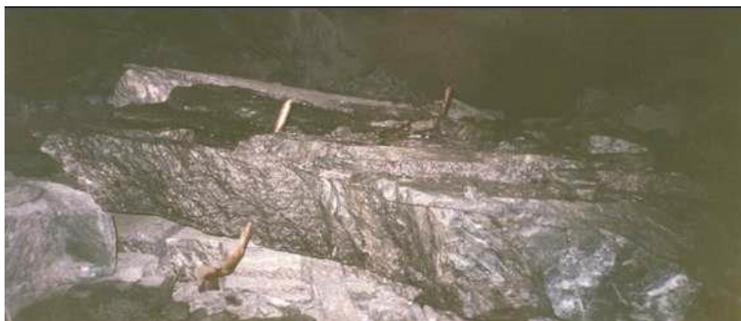
Figure 4 Roof failure caused by over stressing of geological structures
