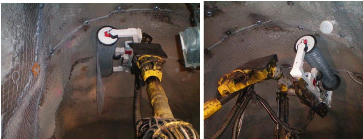
Figure 7 Installation trials in a Western Australian underground mine
