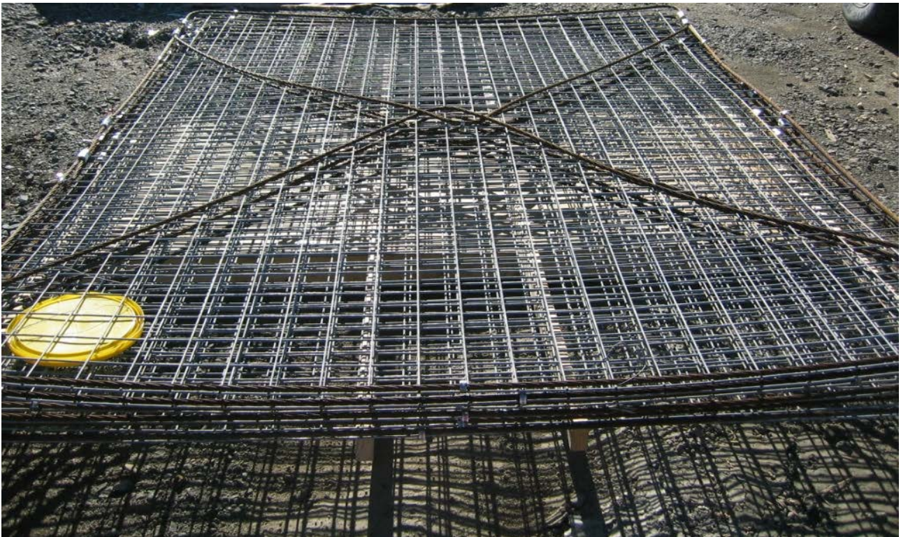
Figure 10 HEA Mesh prior to installation (Potvin and Giles, 2008)
