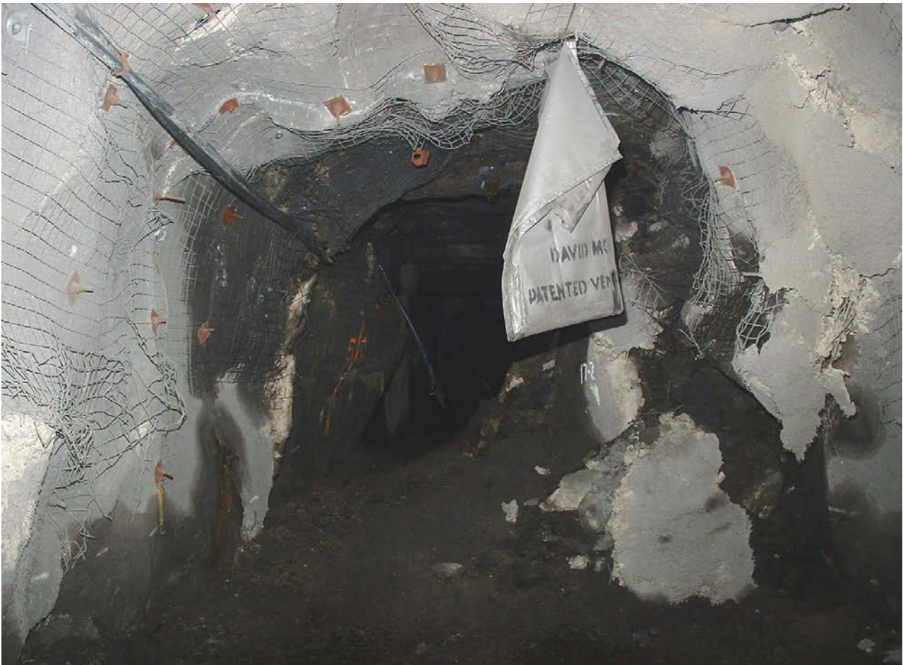
Figure 4 Squeezing ground, 9665 XC17, November 18, 2004
