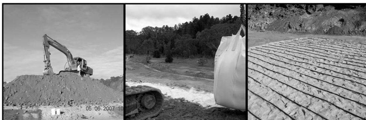
Figure 1 From left to right: construction of test pile; capping of TP1 with EMgO; irrigation system installed on top of a test pile
