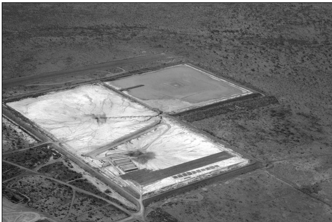
Figure 2 Aerial view of Cells 1, 2 and 3 (taken prior to closure works) with trial works in the foreground
