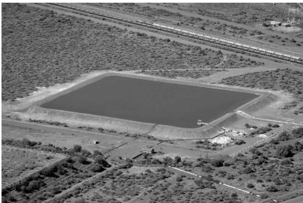
Figure 2 New return water dam
