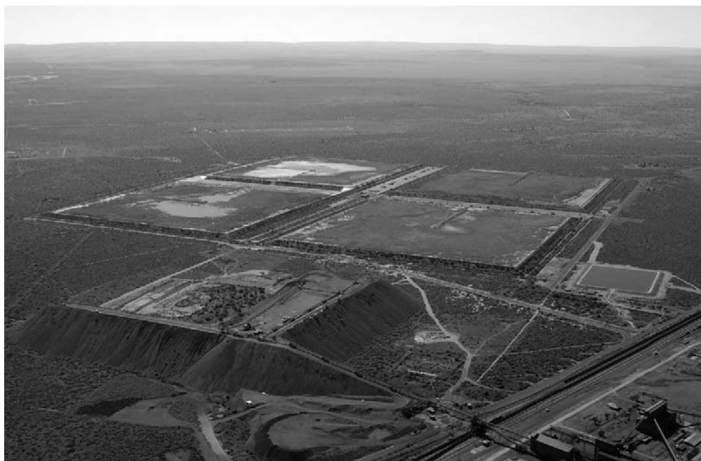
Figure 1 Sishen TSF complex
