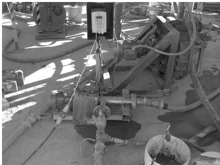
Figure 2 Shear device installation
