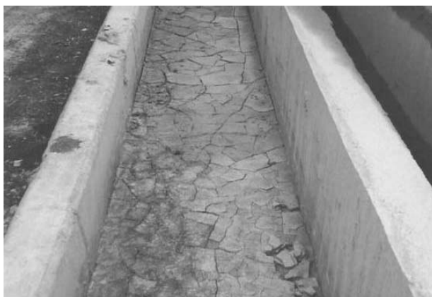
Figure 4 Tailings in the transport channel in a dry state with surface cracking
