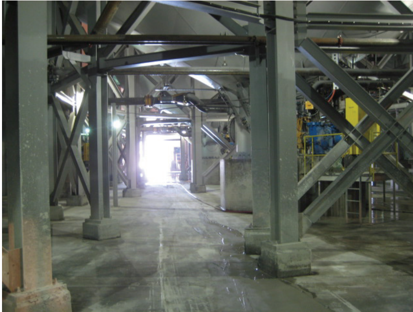
Figure 4 Drive-through access under the CCD circuit
